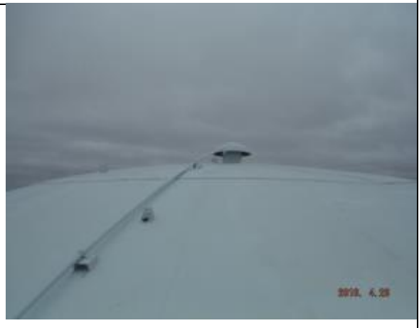
Exterior roof and roof vent
