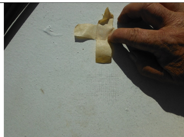
Adhesion test on roof
