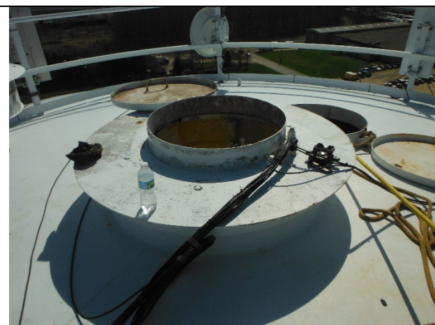
Access tube at exterior roof
