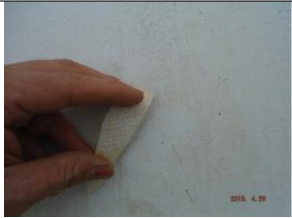
Adhesion test on exterior roof
