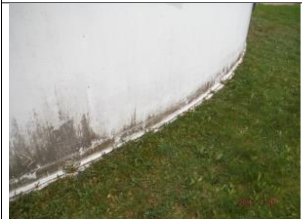
Lower sidewall and foundation
