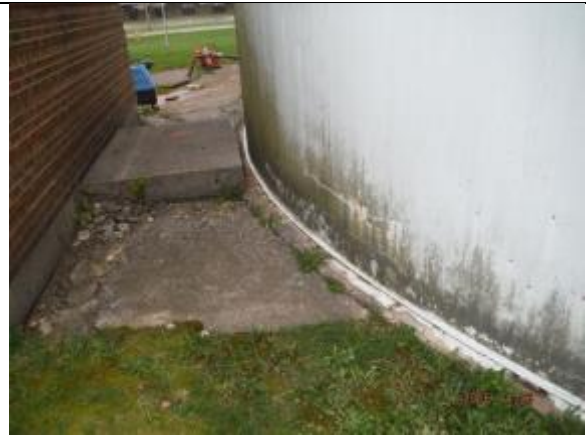
Lower sidewall and foundation
