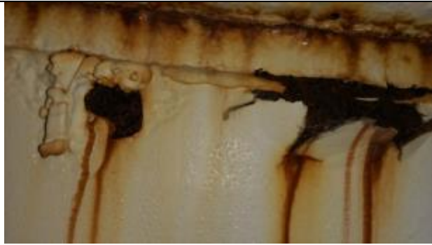
Close up of outer roof sidewall seam
