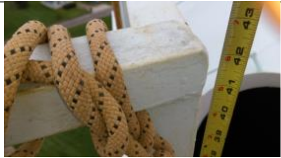
Roof handrail is 42" in height
