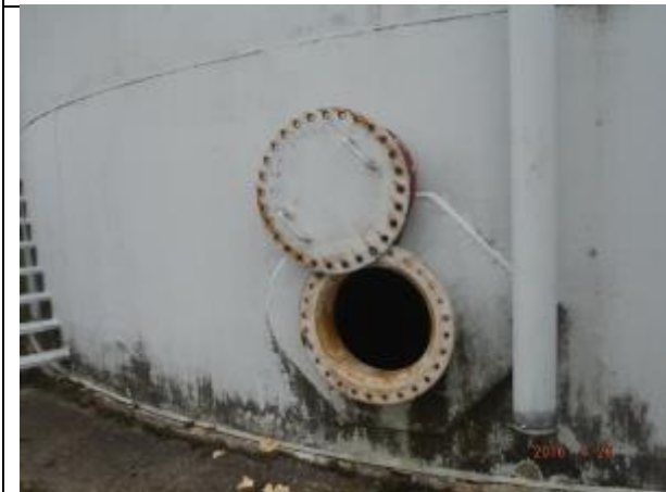
North manway hatch
