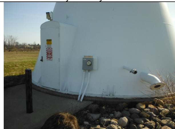
Baseball door and pipes
