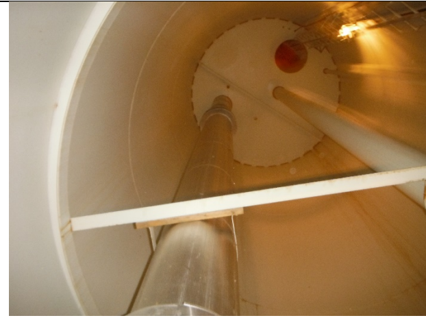
Looking up the interior pedestal
