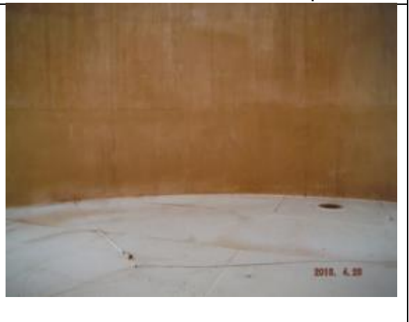
Interior sidewall and floor
