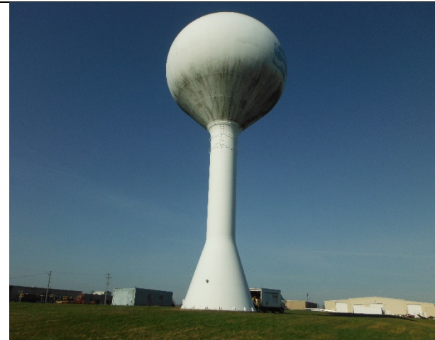
600,000 gallon elevated tank Owned by the City of Owosso
