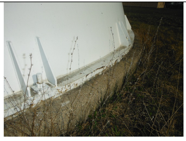
Baseplates and anchor bolts at foundation
