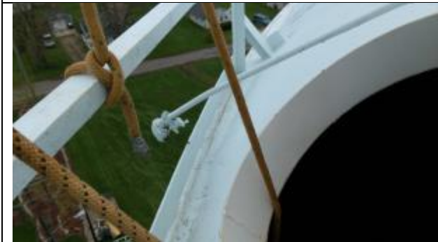
Cut off obsolete conduit on exterior roof
