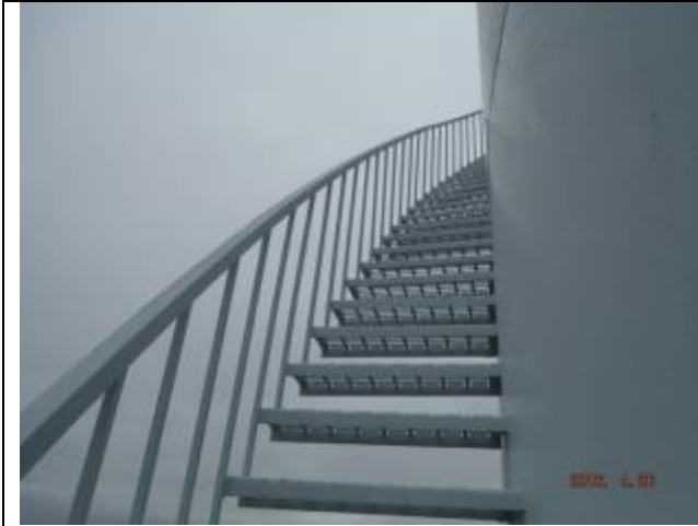
Mid sidewall staircase
