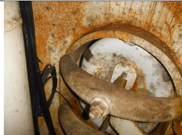
Dry interior access tube manway hatch
