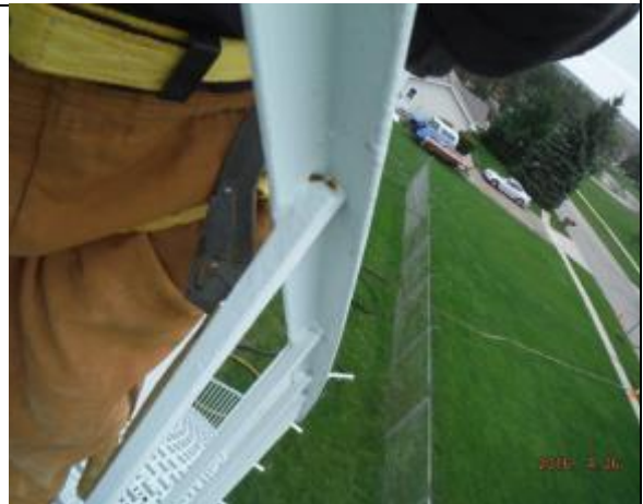
Typical view of bottom side of staircase handrail
