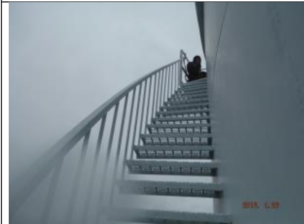
Upper sidewall staircase
