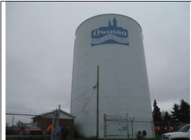
1,250,000 gallon standpipe, Owosso, MI
