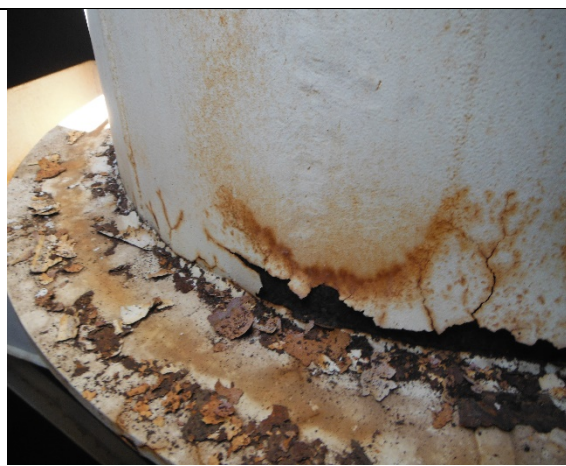
Stiffener on wet interior access tube
