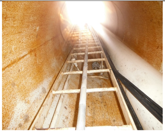
Ladder going up the interior access tube
