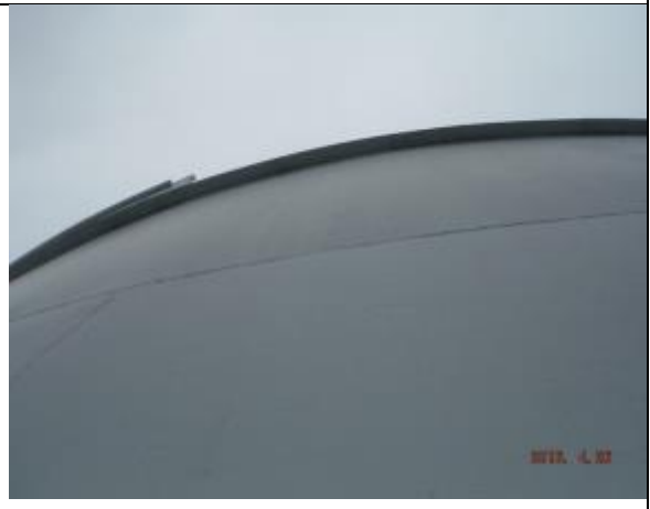
Upper exterior sidewall
