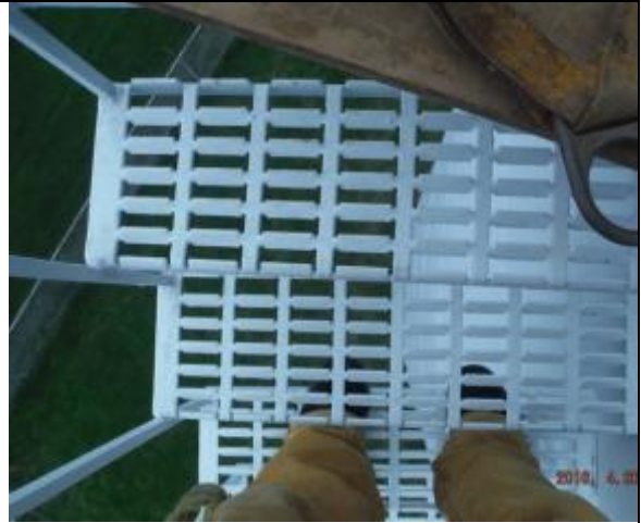
Typical view of steps on staircase
