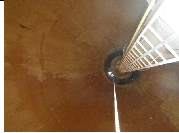
Looking down to bowl from roof
